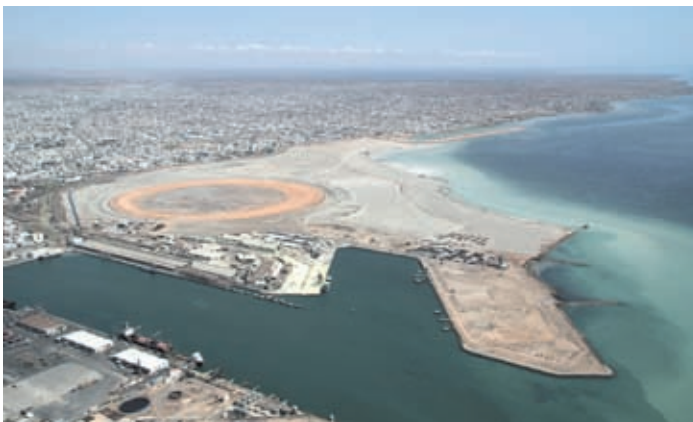
Figure 9. Aerial photo taken at the beginning of the works, during the wet and dry removal of the contamination.
