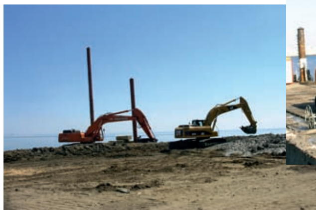
Figure 4. Backhoes excavating the contaminated sediment. Close up of the precision backhoe fitted with an environmental bucket.
