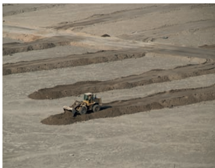
Figure 6. Dry excavation of the contaminated material via bunds.
